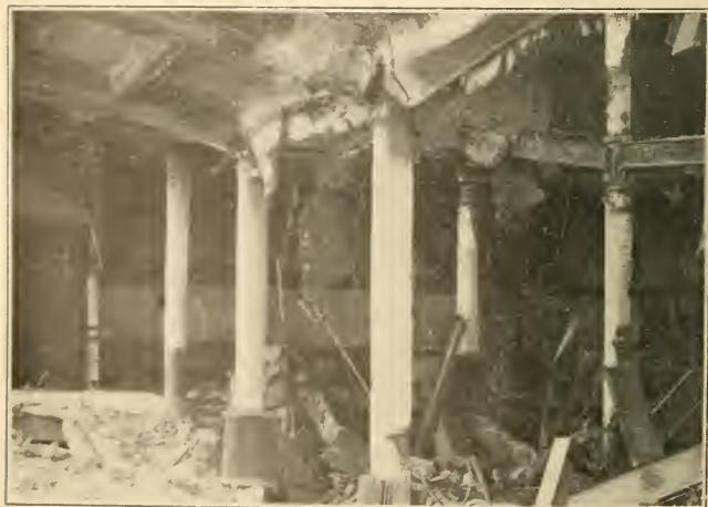
Interior of Sloane Building
